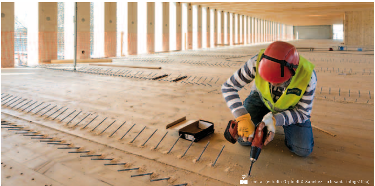
Making of transverse connections
