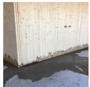
Figure 31. Exposed wall end grain on concrete foundation
