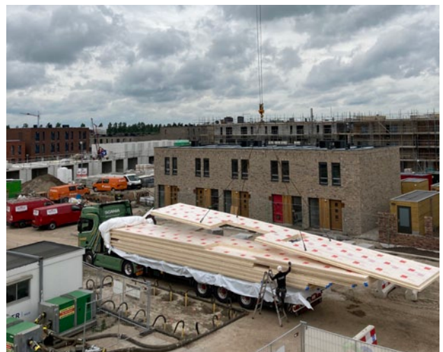
Figure 2. Floor panel lifting
