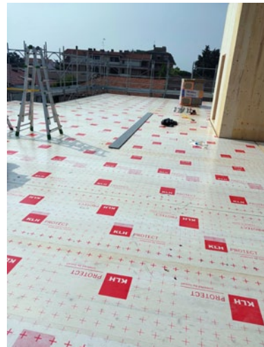
Figure 13. KLH Protect at construction site
