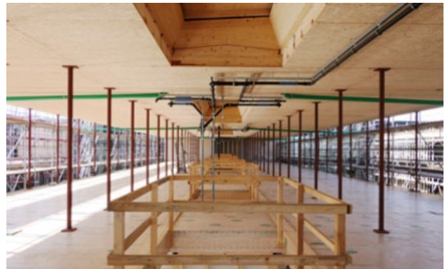
Figure 28. Secured and covered openings during construction
