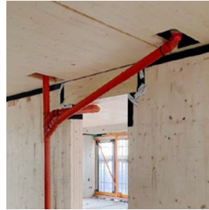
Figure 26. Shaft openings used for temporary drainage
