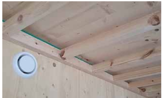
DOUBLE SEPARATION FOR A SUSPENDED CEILING
