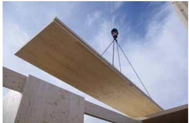
Lifting of KLH® TL panel
