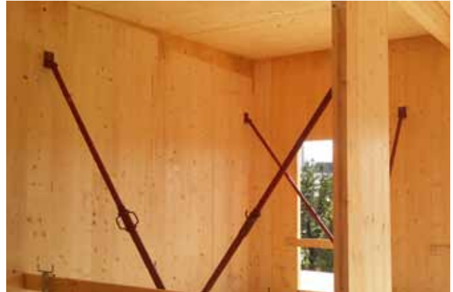
Support during erection in Wiener Neustadt | Austria
