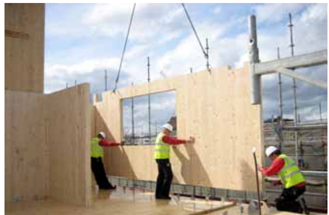
Erection Murray Grove in London | UK
