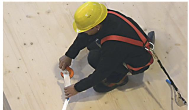
CUT THE LIFTING LOOPS WHEN USING THE VLS SYSTEM
