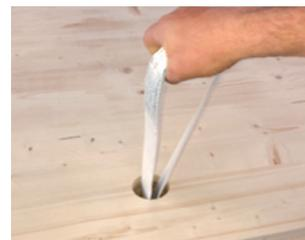
2. Lifting situation with built-in system VLS S
