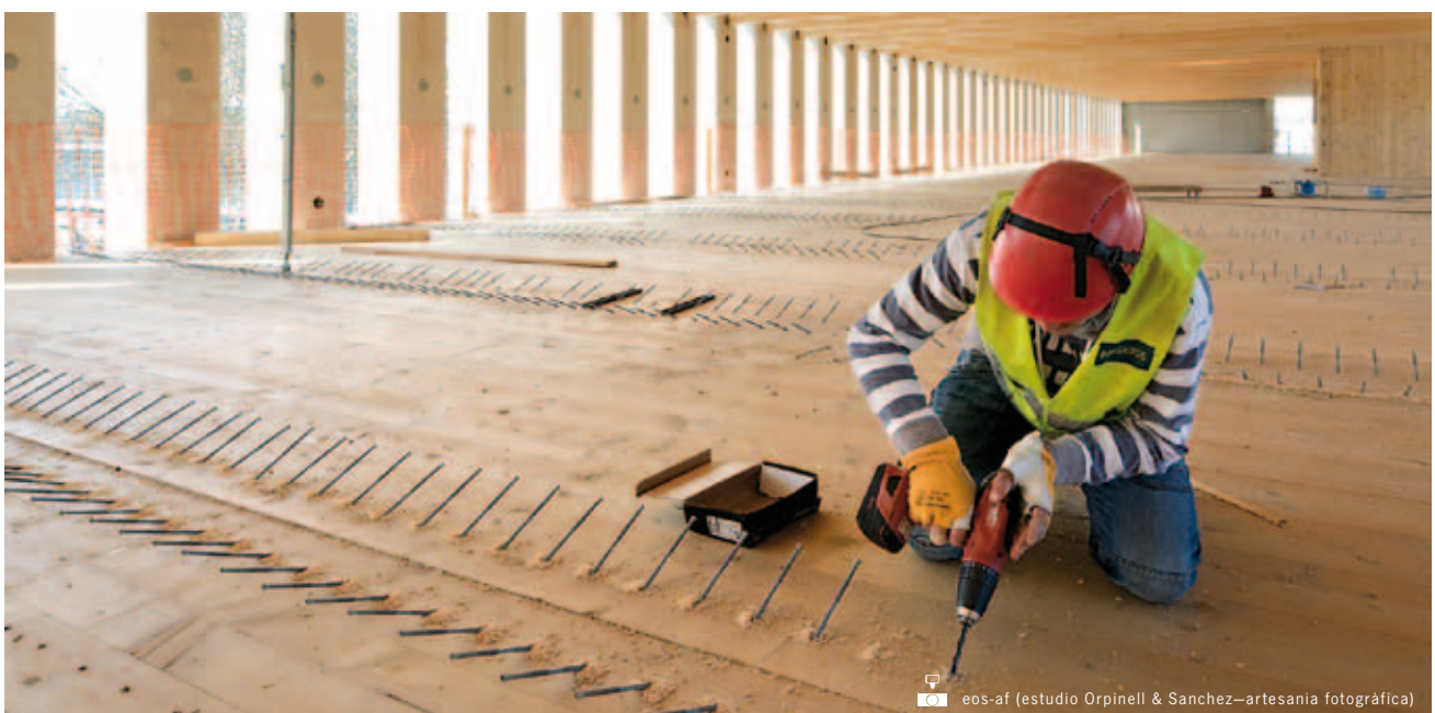
Making of transverse connections
