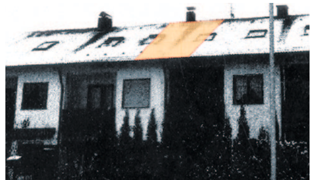
Fig. 9: The same amount of heat is lost per metre of a thermal bridge at the top of the masonry as on three square metres of undisturbed roof area. Weaknesses in the roof area can be easily visually identified in this image from the melted snow.
