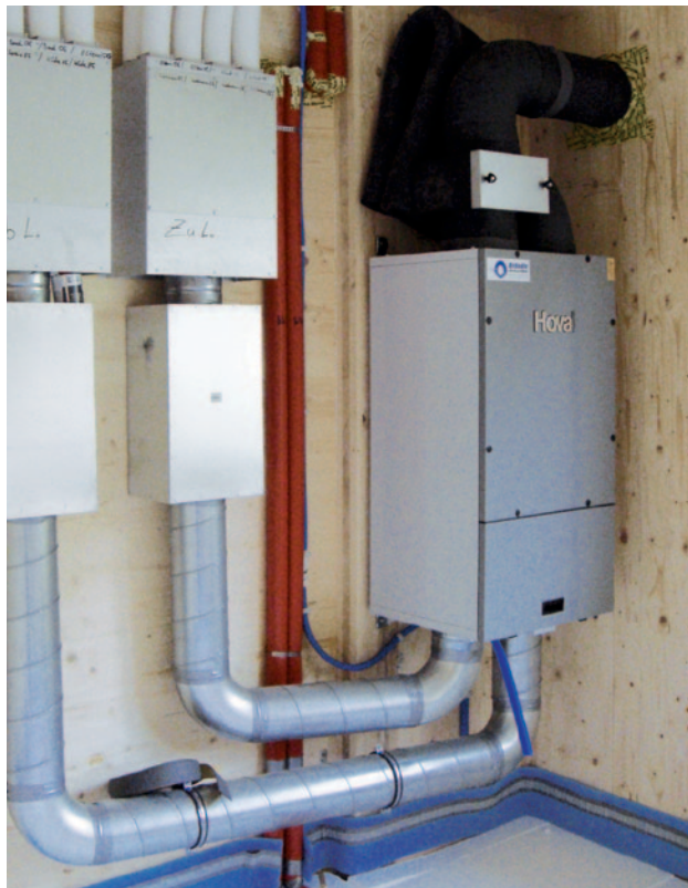
Fig. 13: Mounting of a ventilation system on a KLH® wall [with the kind support of Eberle • d e n k f a b r i k • Dornbirn, Austria].
