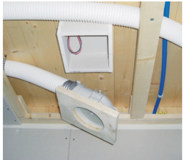
Fig. 14: Running of pipes behind suspended ceiling. System HOVAL [with the kind support of Eberle • d e n k f a b r i k • Dornbirn, Austria].
